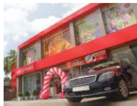
Kaduwela Branch Relocation
